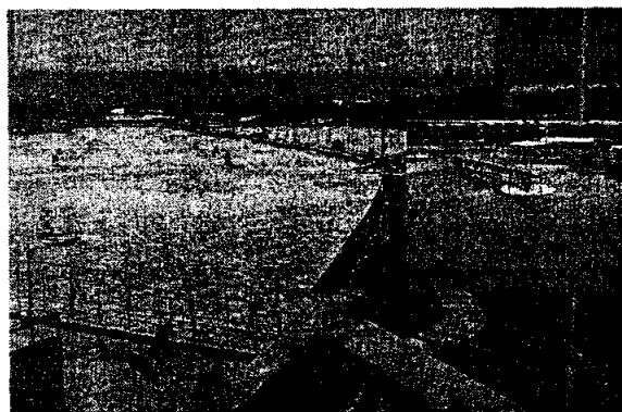
Gambar I.12. Waste water treatment
