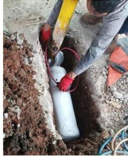
Gambar 4 Cathodic Protection
