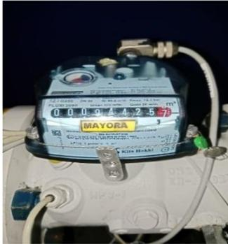
Gambar 5 Turbine Gas Flow Meter G250
