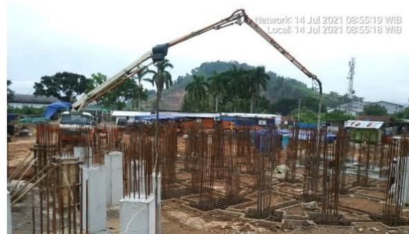
Gambar 5 *System Concrete Pump*
