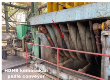
Gambar 10 Fasilitas Heavy Duty Hammer Shredder (HDHS)
