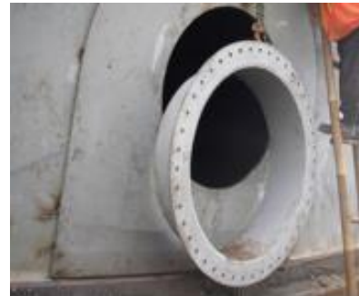
Gambar 8 Fit Up Manhole
