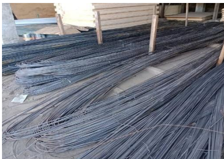
Gambar 4 Pembelian material besi
