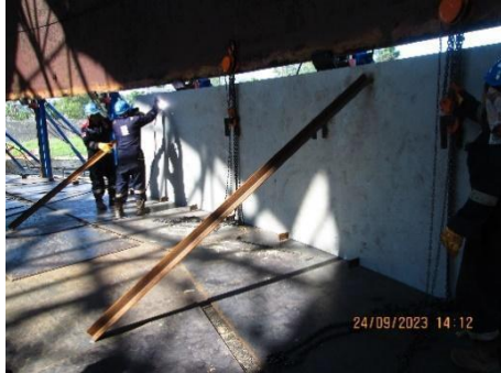
Gambar 5 Erection Plate
