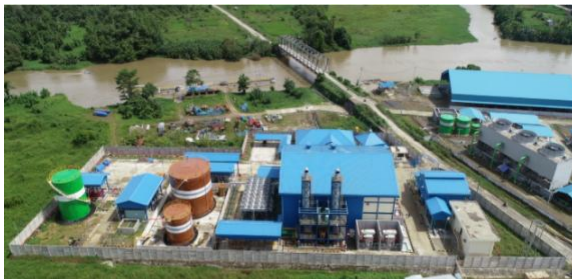
Gambar 2. Foto Plant PLTMG Tanjung Selor 15 MW
