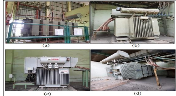
Figure 2. Sample of Transformer (a).150 kV, 63MVA (b). 20 kV,3.15 MVA (c).33 Kv,2.5 MVA (d). 20 kV, 12.5 MVA
